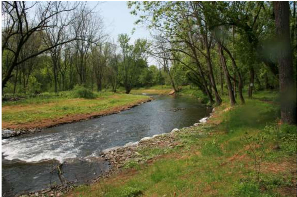
Phase 2 – Middle Reach Post-Construction
