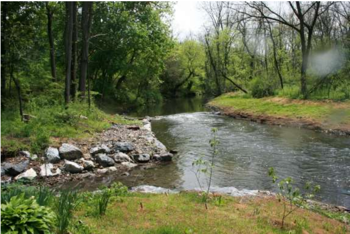
Phase 2 – Upstream Reach Post-Construction
