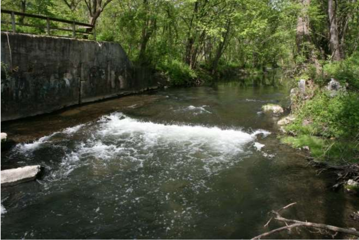
Phase 1 – Upstream Reach prior to removal of Old Mill Dam and Wall
