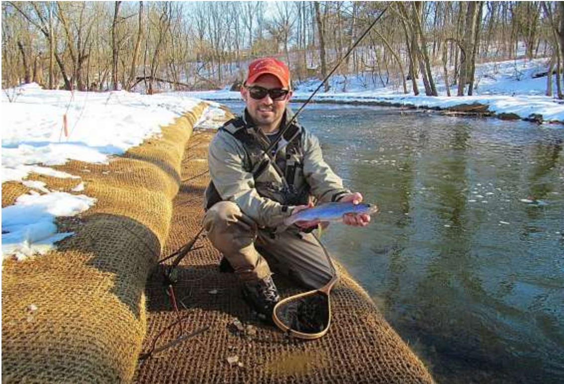
Phase 1 – Downstream Reach March 2015
